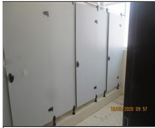
Photo of the sanitary facilities Toilets .JPG
