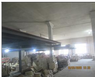
Photo of non-conformity No handrail.JPG
